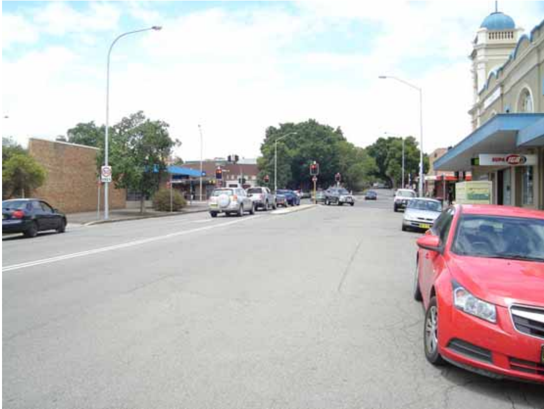
Photograph 5 – Brook Street at Campbell's Corner
