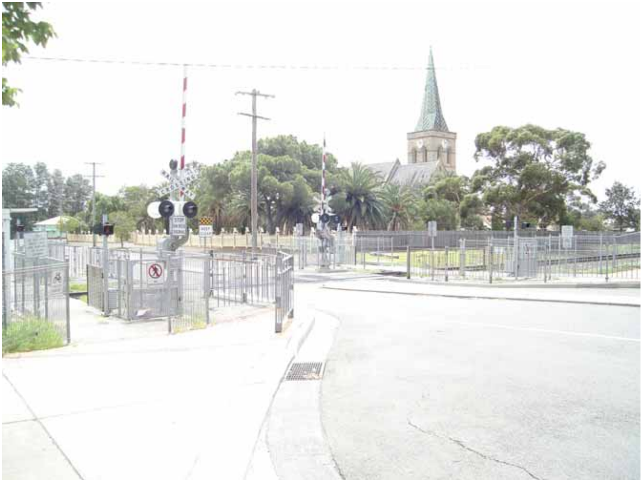
Photograph 8 – Brook Street railway level crossing
