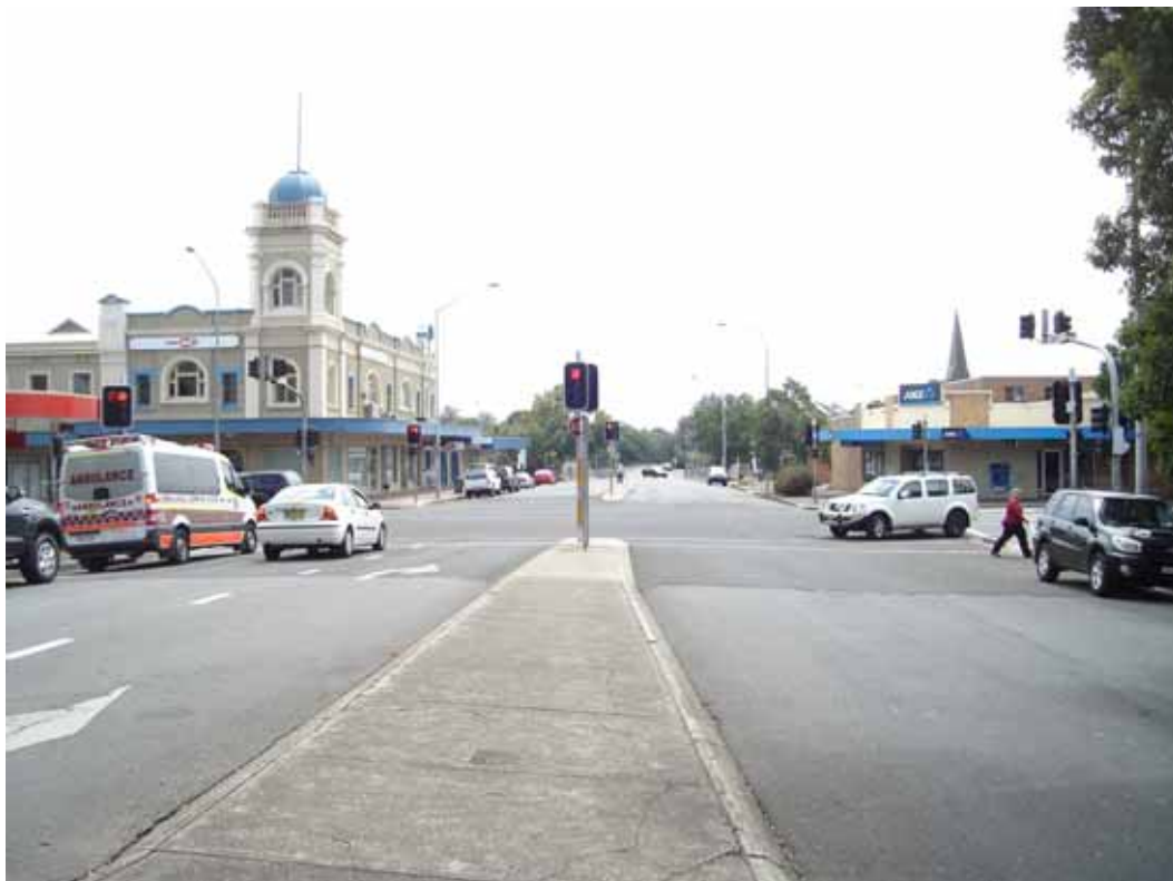
Photograph 6 – New England Highway / Brook Street traffic signals
