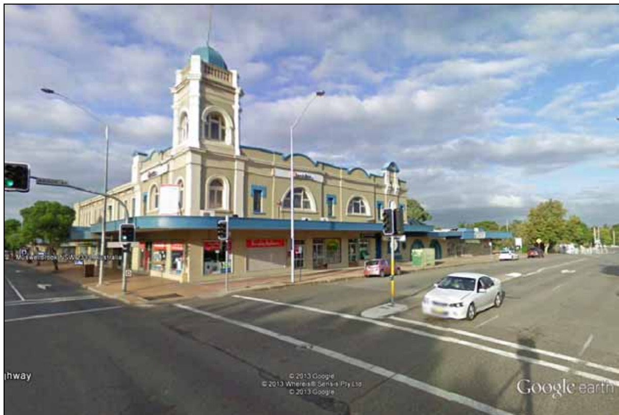
Figure 3 - Campbell's Corner building looking southwest from Bridge St/Brook St intersection
