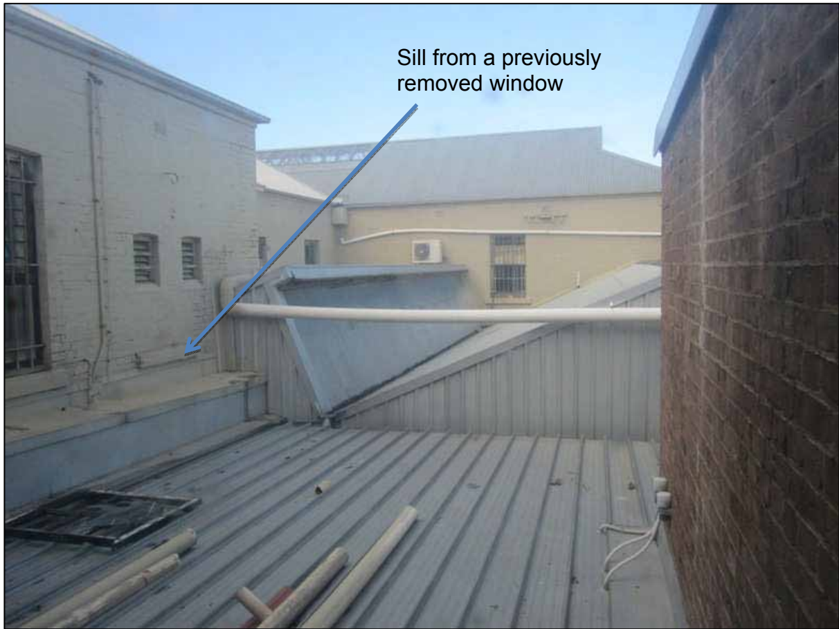
Plate 1: View from the proposed Multi Purpose Room towards the Performance Space wing with the Safe brick wall on the right and the Toilet window and two vents on the left.
