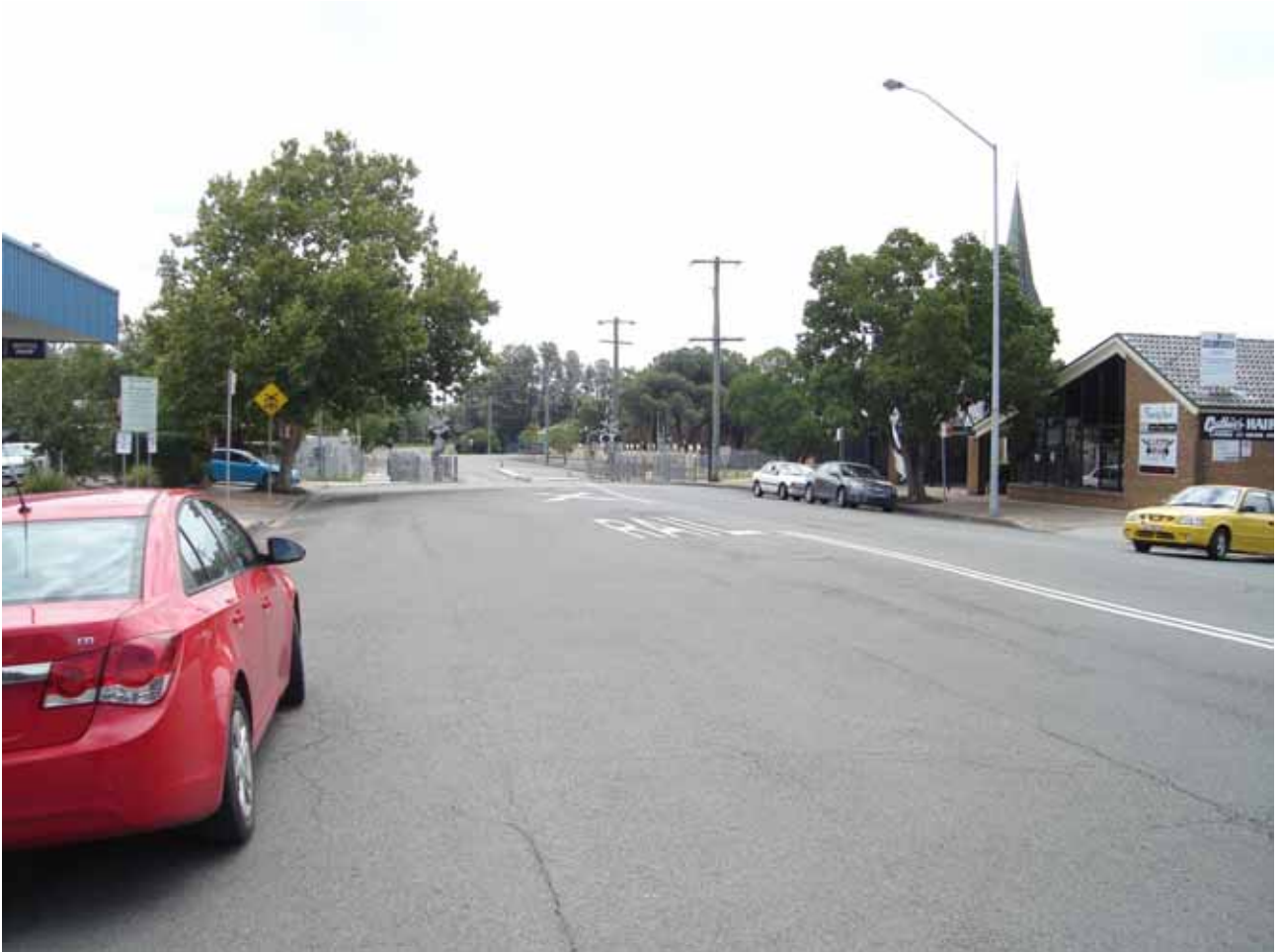
Photograph 3 –Brook Street – looking towards railway crossing
